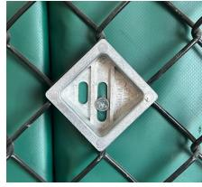
\*\*Chain Link Posts/footings should be designed for the additional weight of the padding. Steel fence ties should also be used. Any damage done to the fence will not be the responsibility of Unlimited Sports Solutions.\*\*
